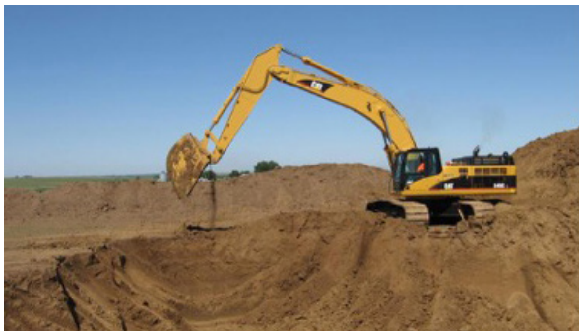
Step 1: Excavation Work Begins
