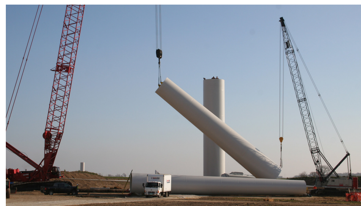
Step 6: Erecting the Tower is Completed
