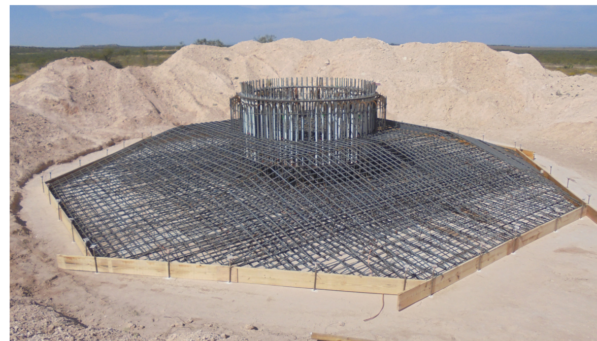
Step 2: Foundation is Started
