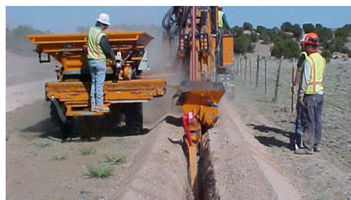
Step 8: Underground Cables are Trenched In
