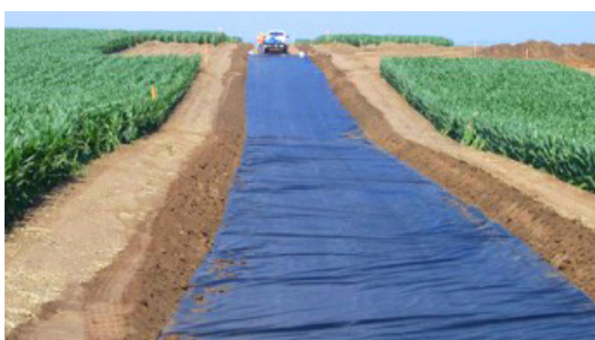
Step 9: Turbine Laneways are Completed
