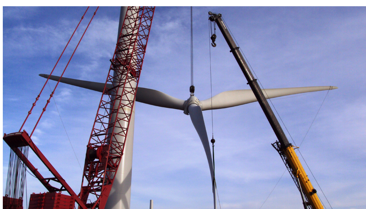
Step 7: Nacelle & Turbine Blades are Attached
