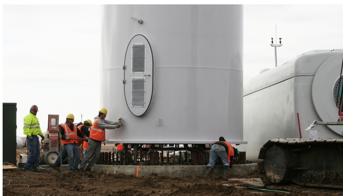
Step 5: Base is Attached to Tower Foundation
