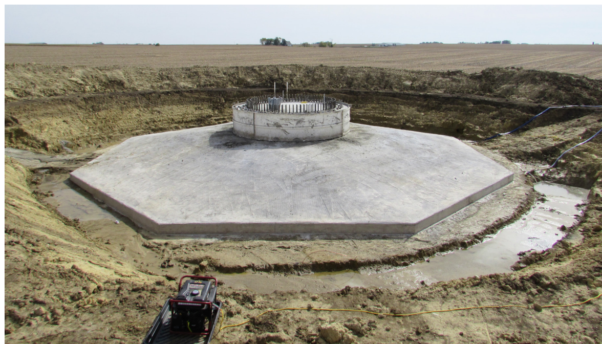
Step 3: Concrete is Poured
